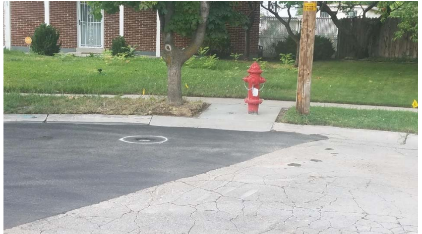
Figure 4: New fire hydrant after installation located at 4471 W Fassio Circle.
