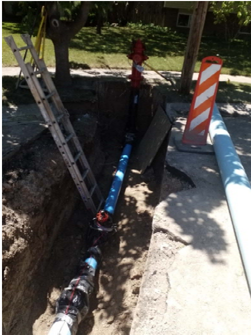
Figure 3: New fire hydrant during installation at 4471 W Fassio Circle.
