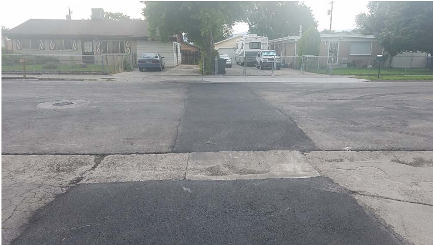
Figure 5: New road asphalt patch on 4400 W Fassio Circle.
