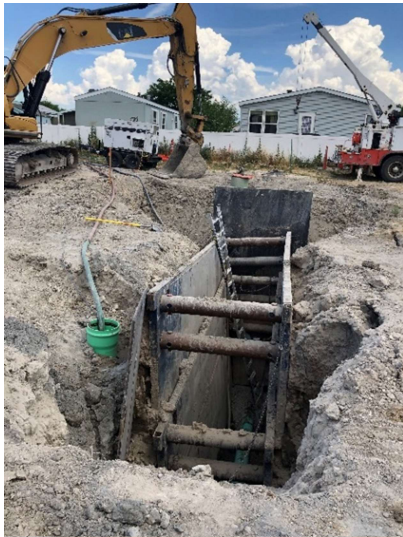
Fig. 5: Installing first section of pipe
