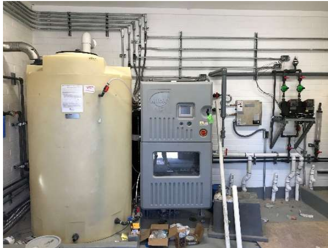
Fig. 4: New MIOX Generator Installation
