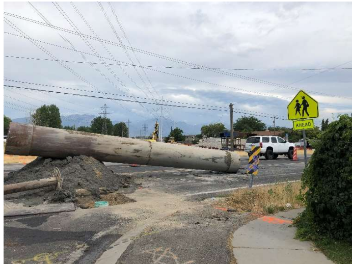
Fig. 6: Casing used for dewatering well
