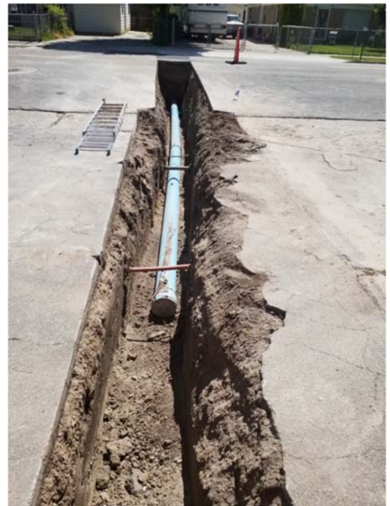
Figure 6: New pipe installation located at 4400 W Fassio Circle.
