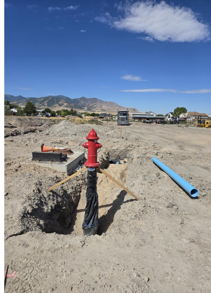
Fire hydrant installed
