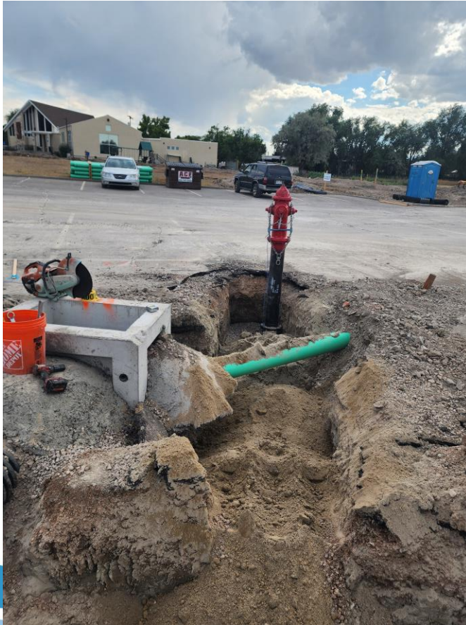
Fire hydrant installed
