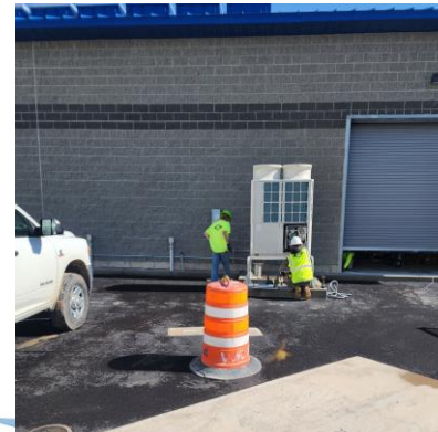
HVAC Unit Installation
