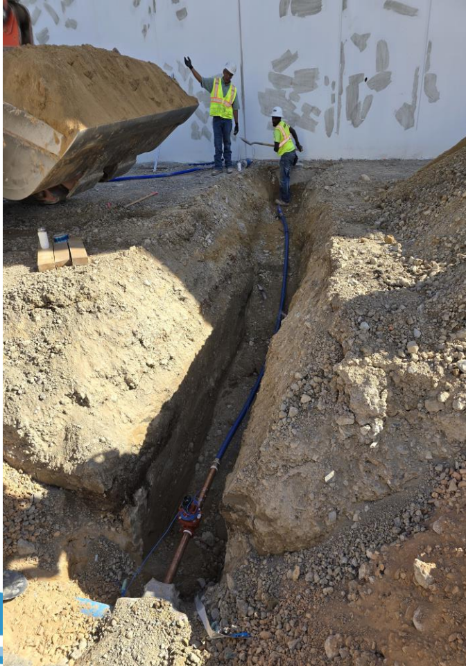
2" water lateral and valve into building
