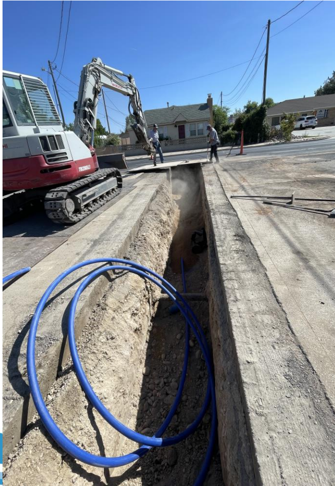
2" water lateral install
