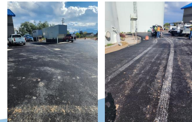
Asphalt Installed Near Building, Generator, and Tanks
