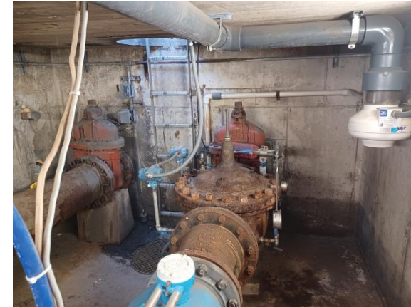
Existing Condition of Vault
