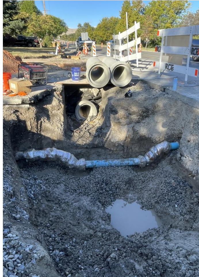
6" water main loop for storm drain conflict
