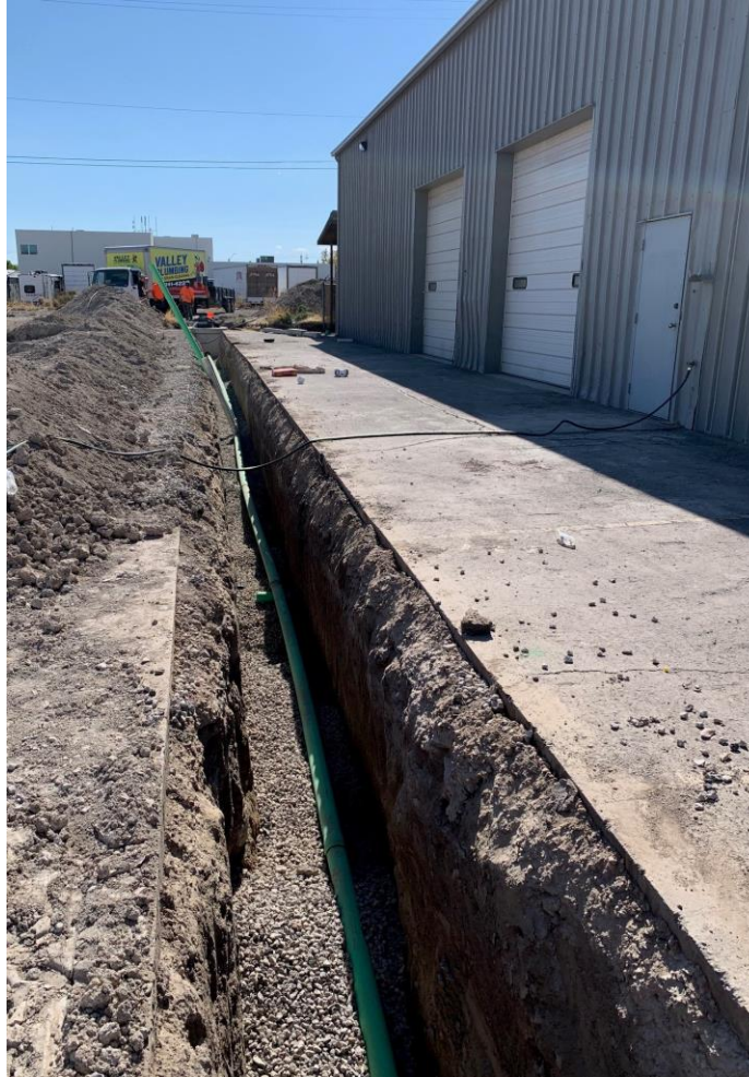
4" sewer lateral install
