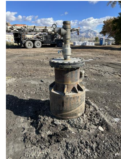
Well Capped Off
