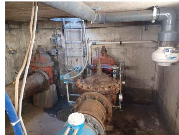
Existing Condition of Vault
