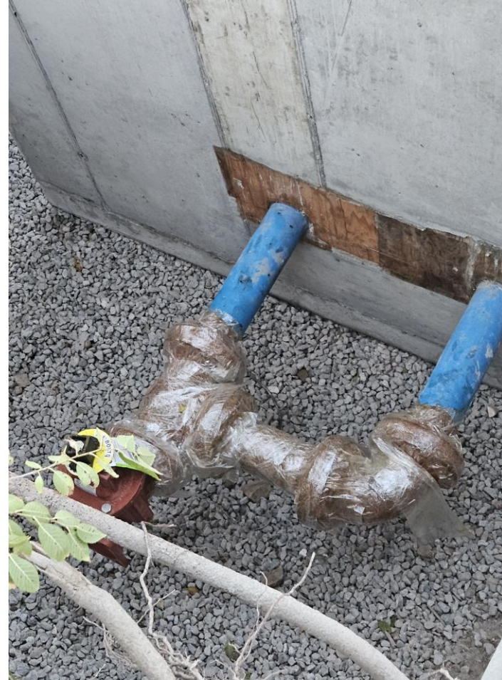
4" meter vault with epoxy and wax wrapped fittings
