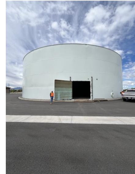
Acord Reservoir Tank
