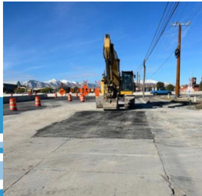
Temporary asphalt patch
