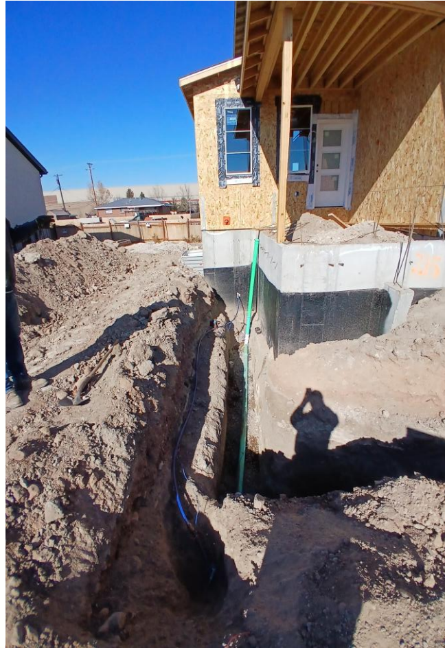
¾" water lateral and 4" sewer lateral Install
