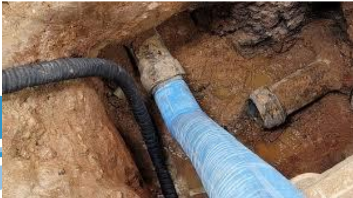
CIPP liner being installed into a sewer main
