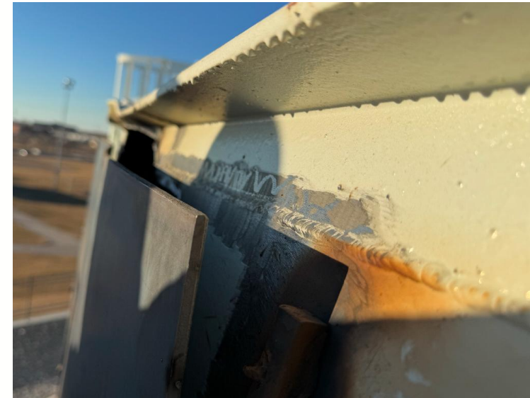
Top Portion of Reservoir Prepared for Welding
