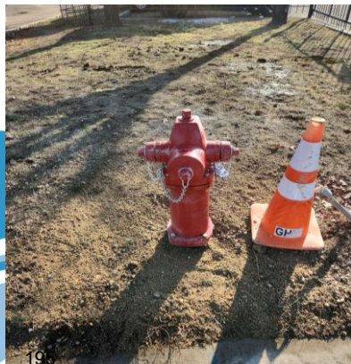
New hydrant @ 4765 W 3500 S
