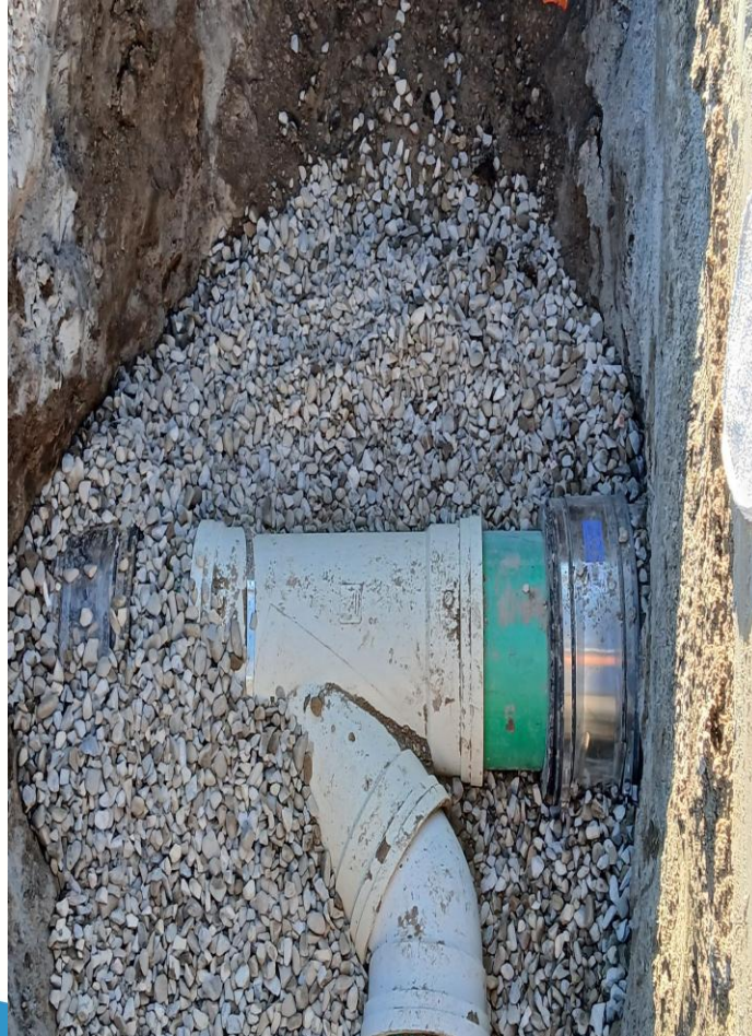
8" sewer lateral installed with new main connection
