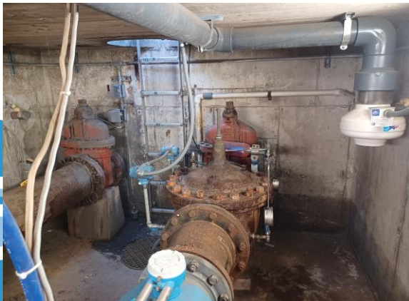
Existing Condition of Vault
