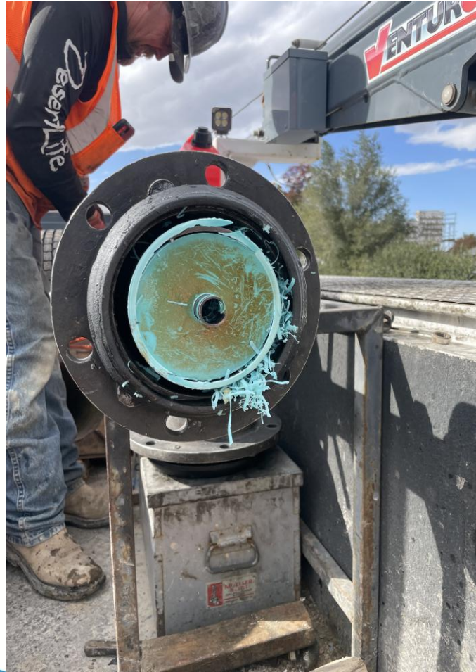
8" fire line and PVC coupon from hot tapping process
