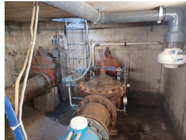
Existing Condition of Vault
