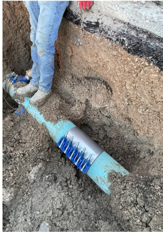
1.5" water lateral connection
