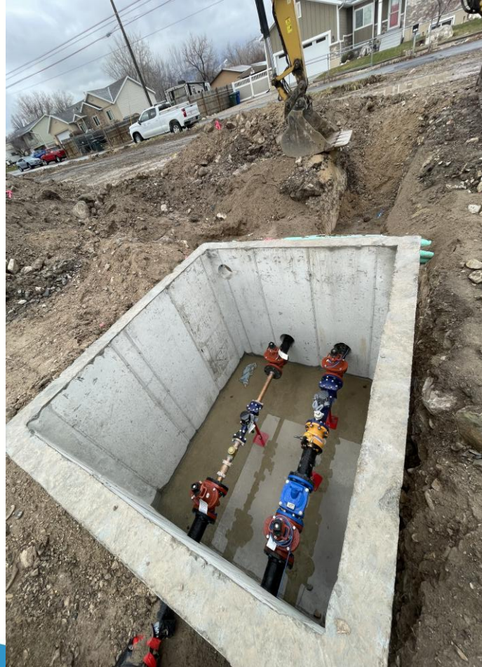
4" meter vault and 10" double check detector assembly
