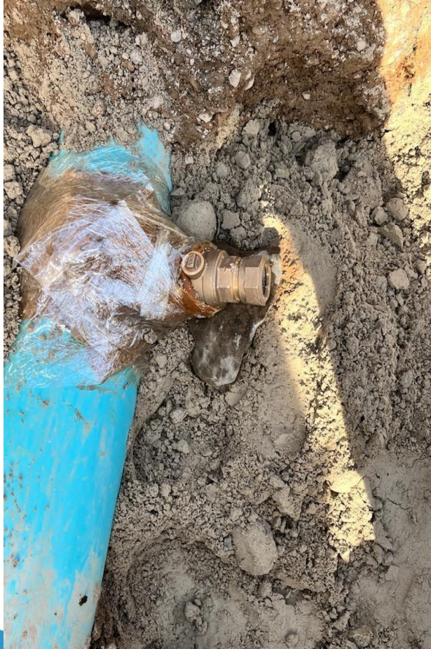
1.5" water lateral connection
