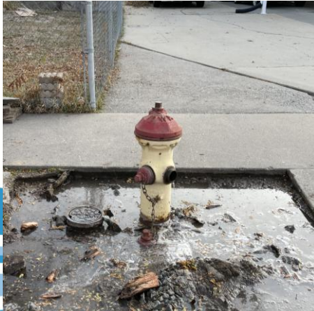
Hydrant on Mock Orange Drive prior to new installation
