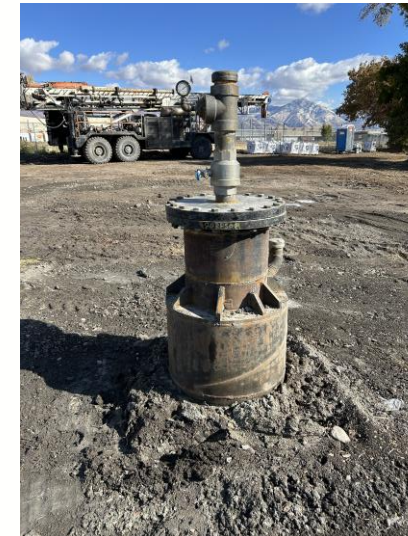
Well Capped Off
