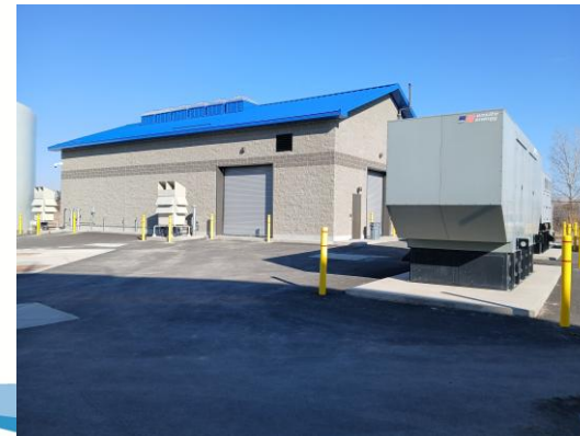
Kent Booster Pump Station Building
